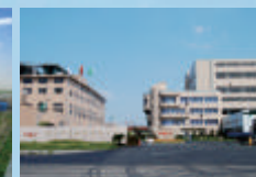
TBR Plant in Xiasha
